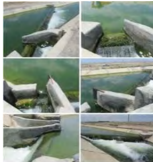
Figure 4.30 Performance of the built structure after the operation with discharge
