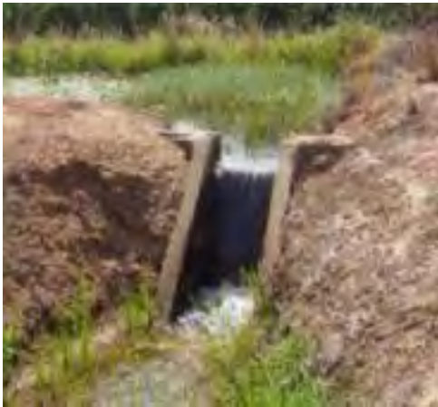
Figure 4.2 Newly installed channel regulator structures
