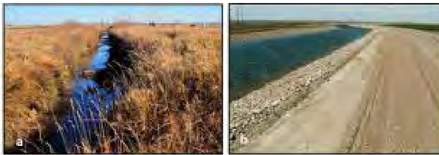
Figure 4.9 Unrehabilitated (a) and (b) rehabilitated canal
