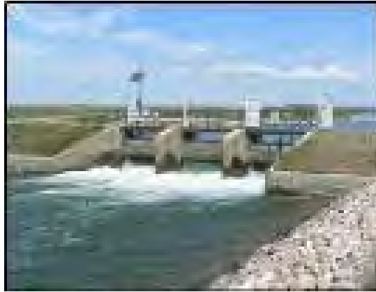
Figure 4.8 Automated check/drop structure
